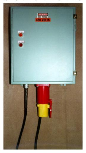
Standard or Custom Packages to provide railway passenger cars with power from station, shop, or other utility power while stopped for maintenance or layover, from
