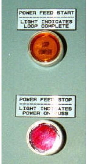
Simple, easy to use control button system with indicator lights for system status.
