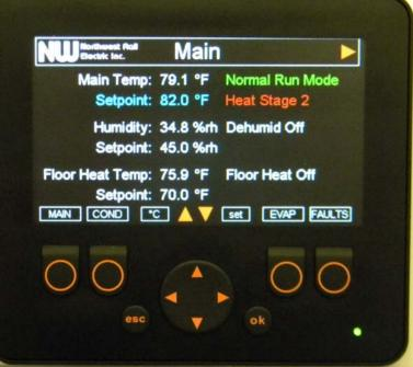
Main HVAC system display screen (above) and a small portion of the technical details and system status and fault monitoring that is available (below). System includes detail displays for condenser and evaporator status and many other items helpful for diagnosis.
